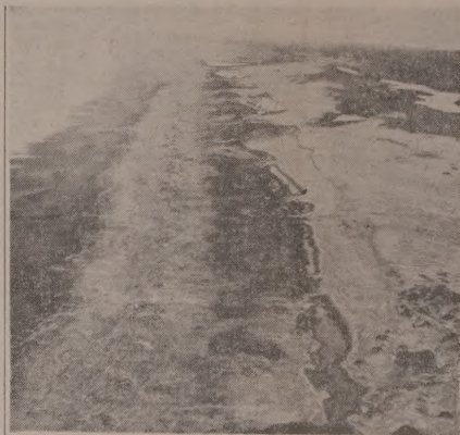
"Before" picture shows Surf Pines area in 1937 at start of reclamation project. Wind and sand had gouged gaps, allowing sand to invade and cover lush meadow land, fill lakes and threaten resorts. Sand was crossing neck of land, piling into the Columbia River, threatening navigation.
