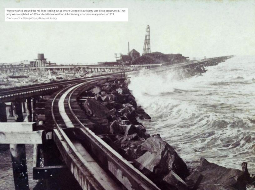
during winter's wild weather, and it was one which that winter uproar would "unravel," bashing boulders around, weakening the structure. Summer's work began with repairs to last fall's work.
